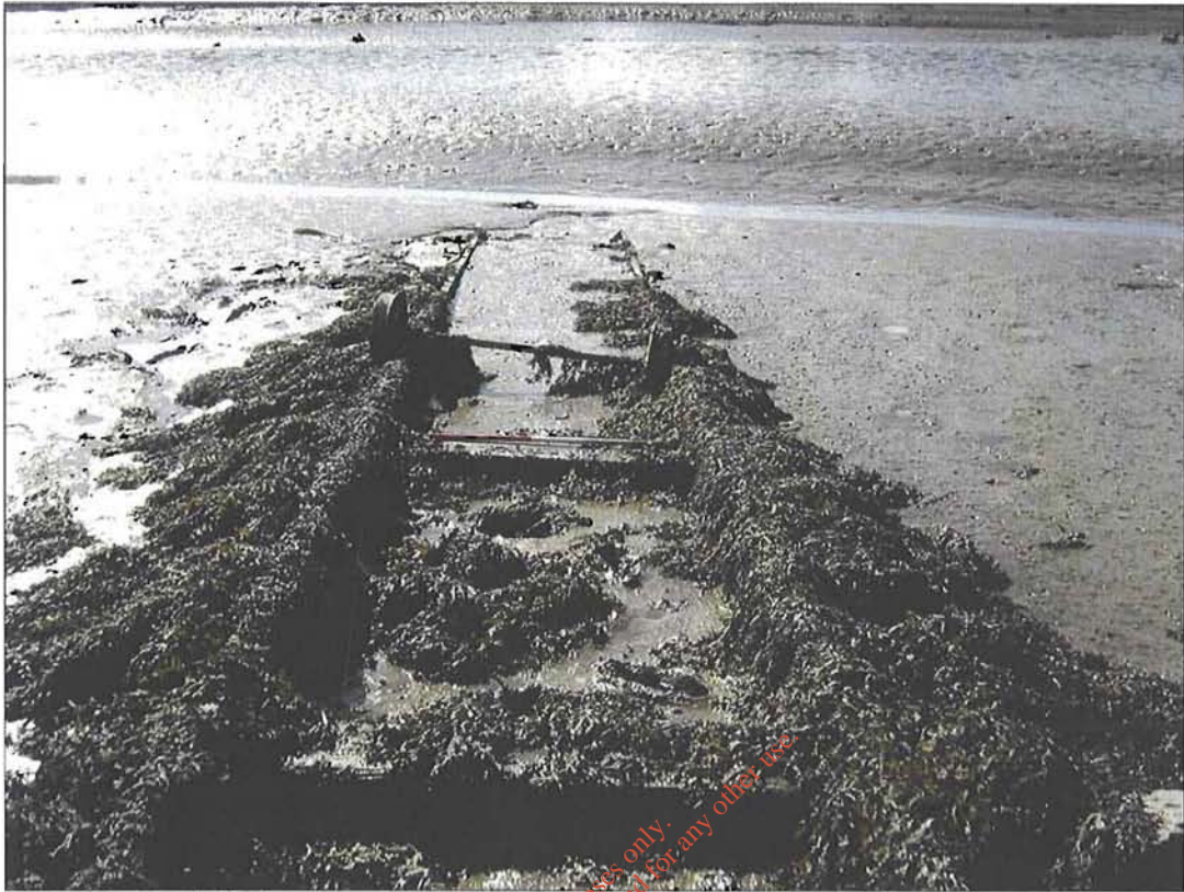
Plate 29: South-facing view of iron-trackway for boat-trolley/ launch located c. c.1520m along proposed pipeline route (see Figure 7 for location), 1m scale.
