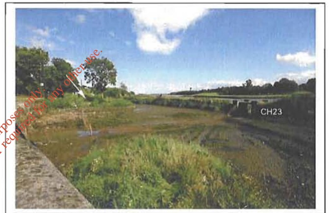
Plate 3.43. Proposed location for major pumping station at Raffeen/Strawhill, from northwest
