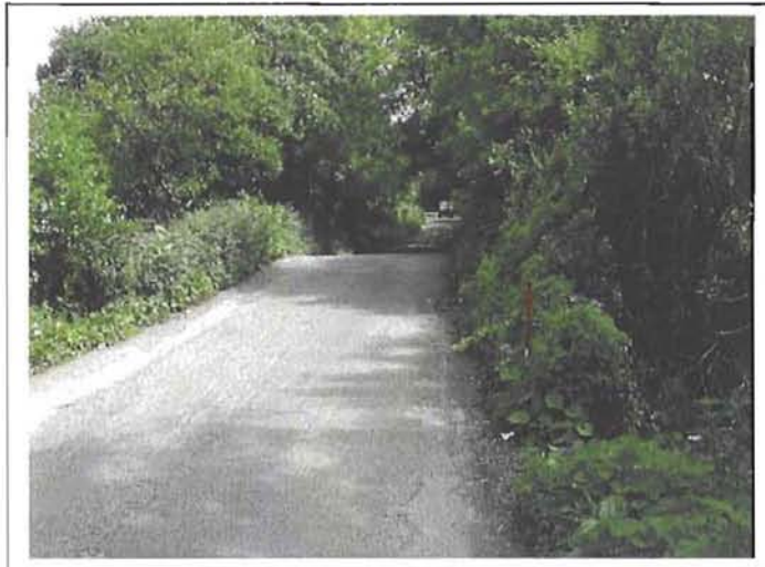
Plate 3.12. View southward over 'Dandy bridge' in Kilnagarry
