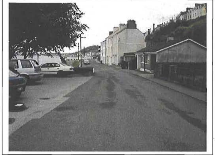
Plate 3.30. Pipeline along roadway at east side of Cobh, from east
