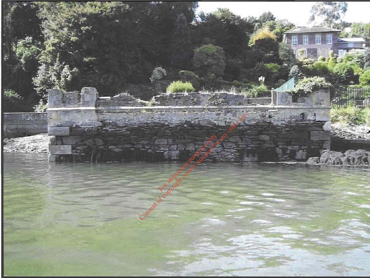
PLATE 3.8.4 WEST-FACING VIEW OF DOWNSTREAM (SOUTHERN) MASONRY FACADE FROM THE SOUTH WING OF THE ROYAL VICTORIA BATHS
