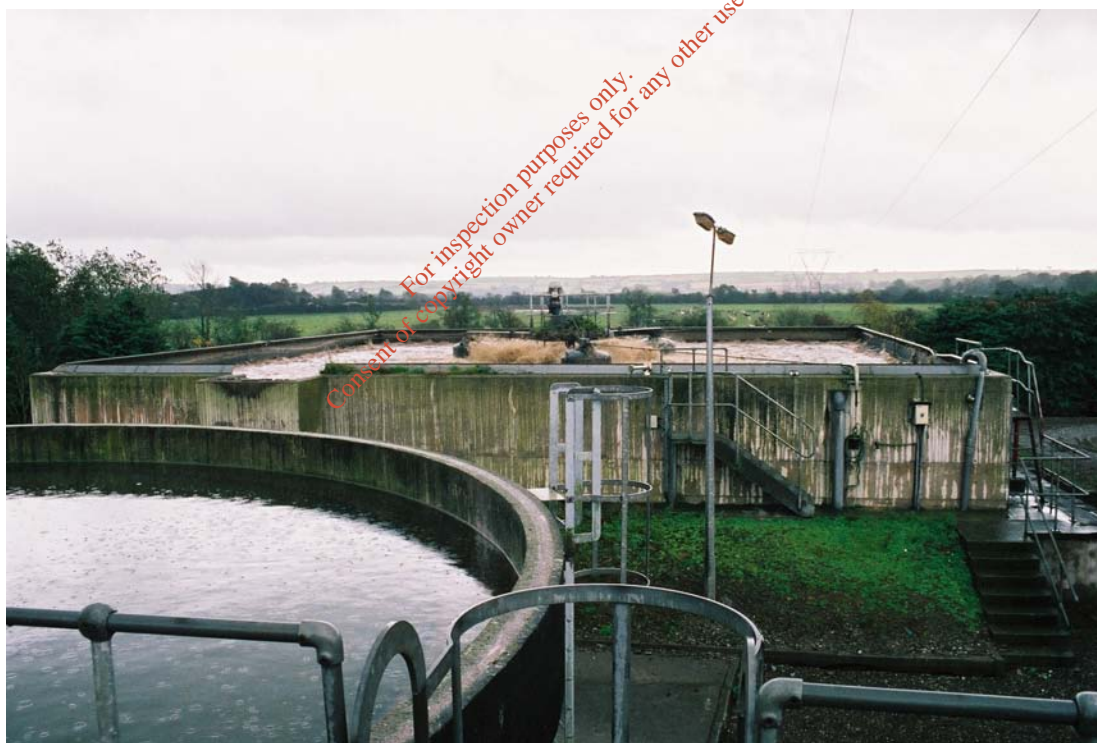
Photograph 1.1 – Balancing tank at the Carrigtohill works
