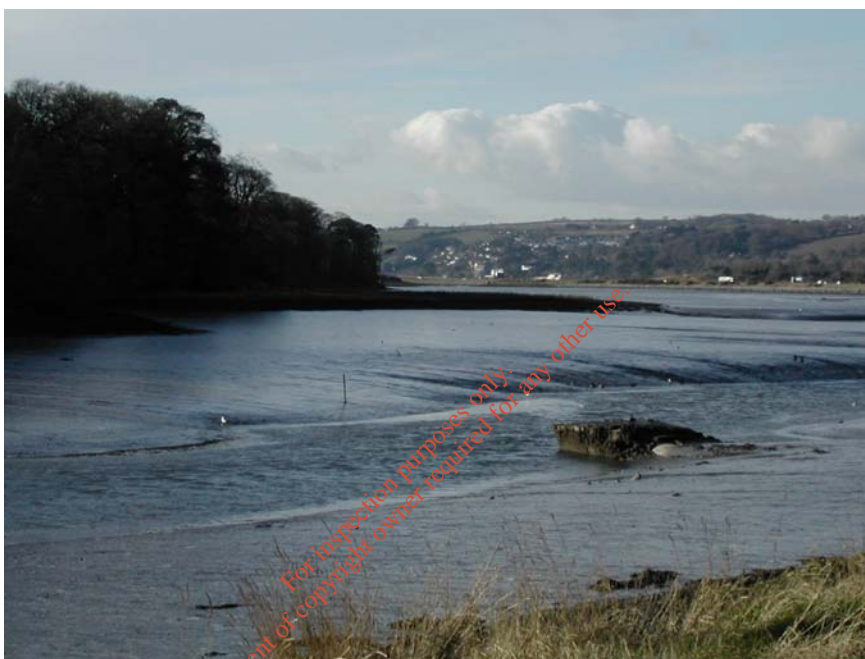
Photograph 4.1 Existing Outfall to Slatty Waters
