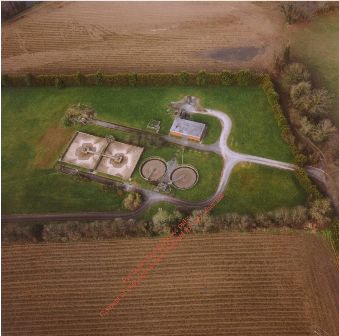
A1.2 Mallow Sewage Treatment Works viewed looking north
