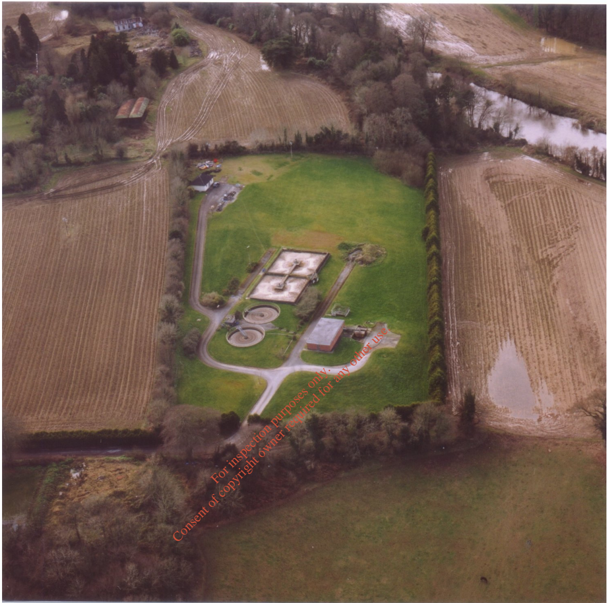
A1.3 Mallow Sewage Treatment Works viewed looking west
