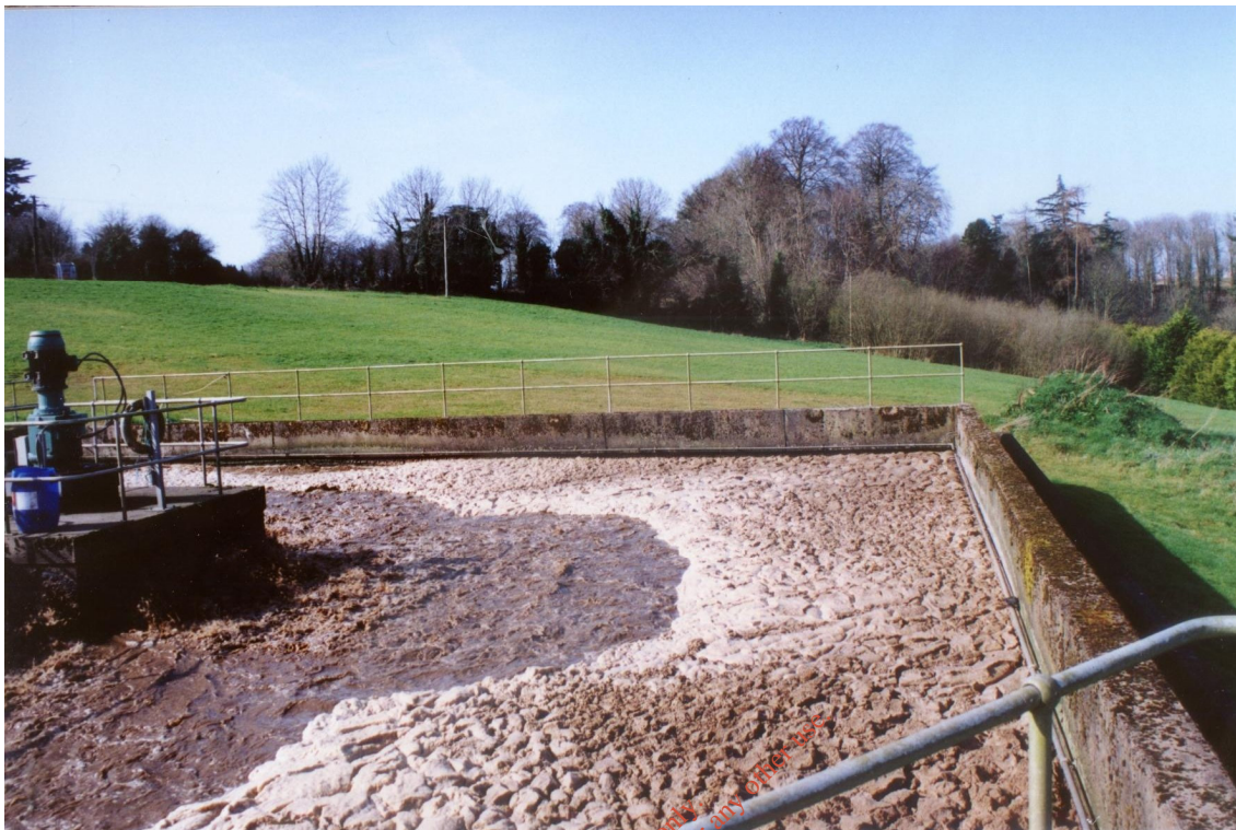
Figure 2.6 Aeration Tank with green space in the background
