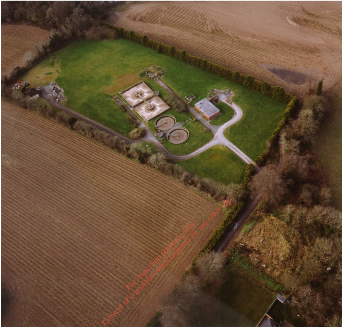
Figure 2.2 Aerial Photograph of Mallow STW viewed looking north-west For further photographs see Appendix 1.
