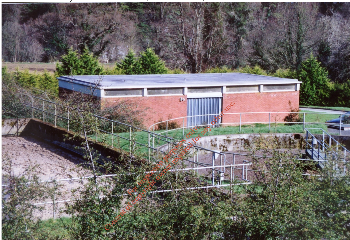
Figure 2.3 Aeration and Clarifier Tank with Sludge Dewatering Building behind
