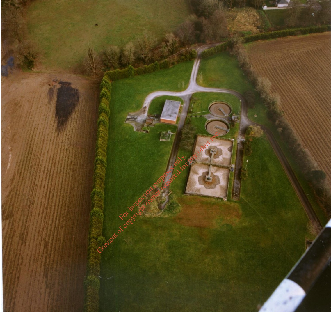
A1.1 Mallow Sewage Treatment Works viewed looking east
