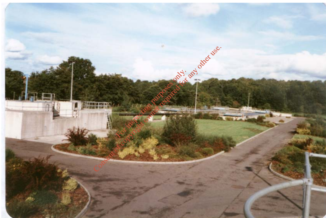
Figure 2.5 Fermoy Sewage Treatment Works (photograph taken just after construction)
