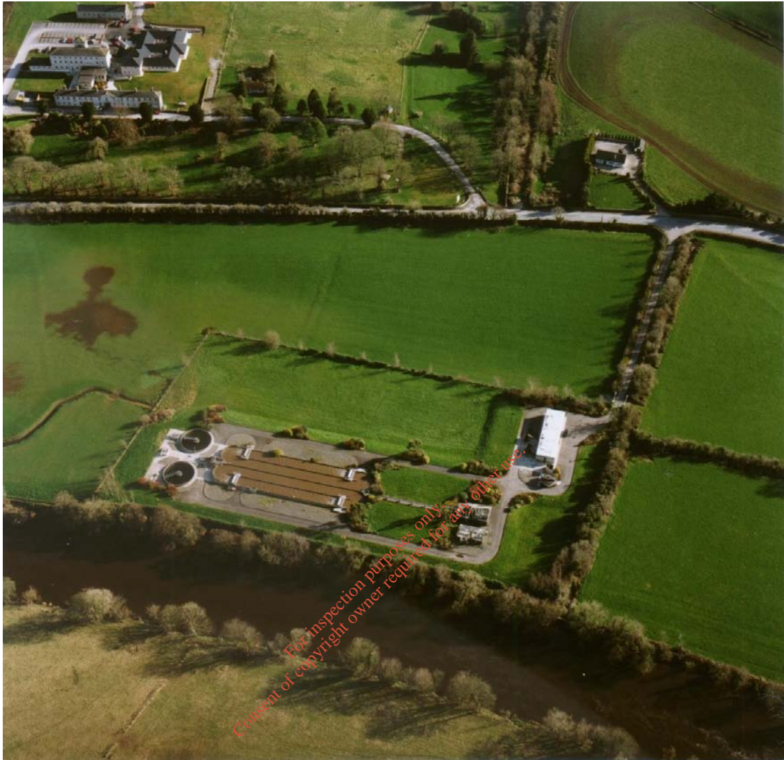
Figure 2.3 Aerial Photograph of Fermoy STW viewed looking south
