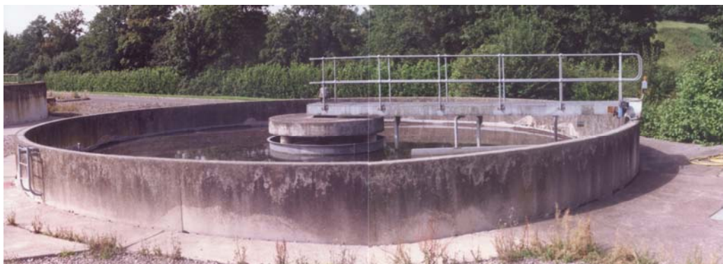
Figure 2.4 Existing Clarifier Tank
