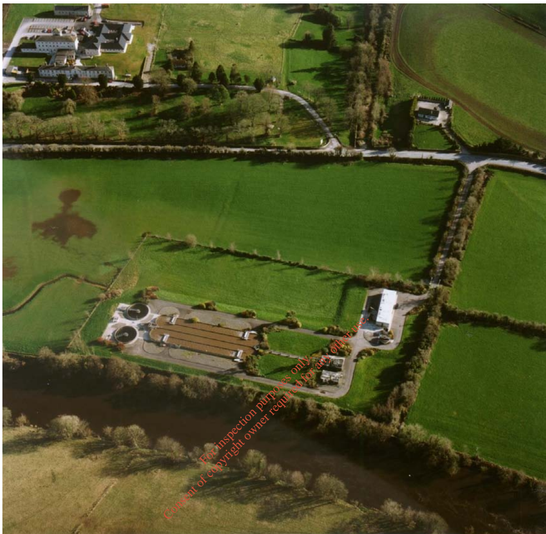
Figure 2.3 Aerial Photograph of Fermoy STW viewed looking south
