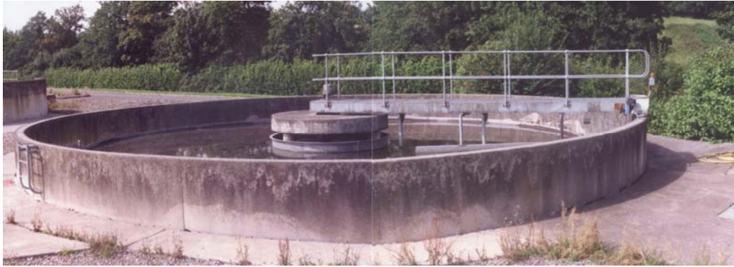
Figure 2.4 Existing Clarifier Tank
