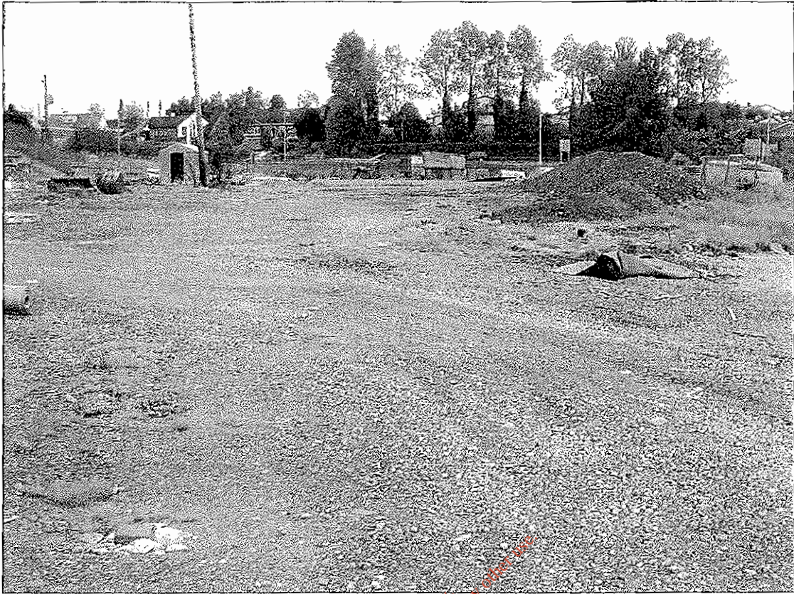
Plate 7: Location of proposed blower building, administration building, inlet works and storm tanks, currently under stone gravel and used for storage, looking south.
