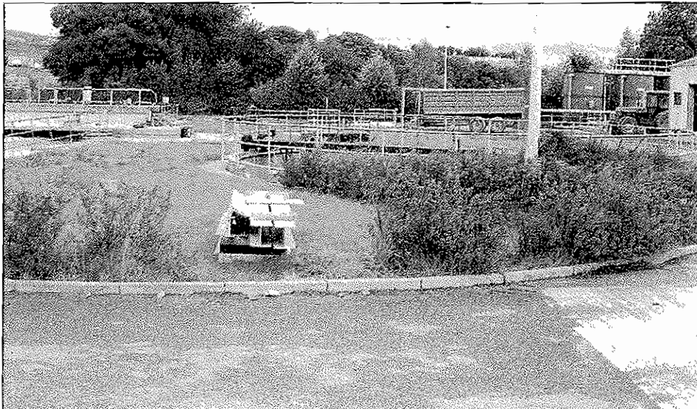
Plate 6: Oxidation ditch, settling tank and sludge chambers to be redeveloped.
