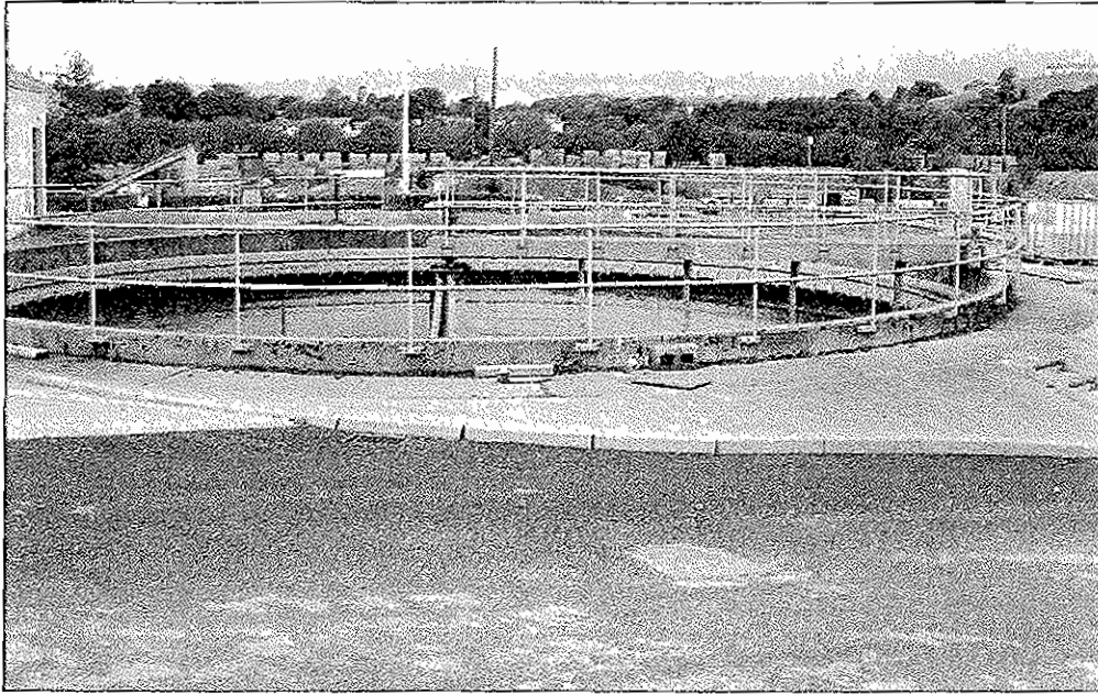
Plate 4: Existing storm water tank with concrete surrounds, looking west.
