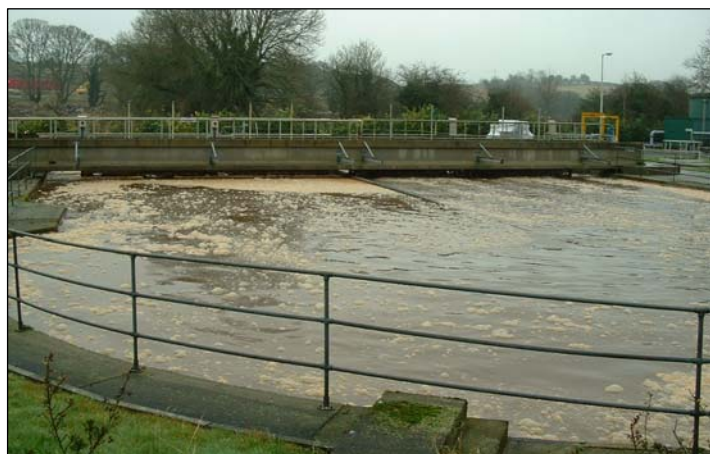
Photograph 3.3 – Oxidation Ditch No.1
