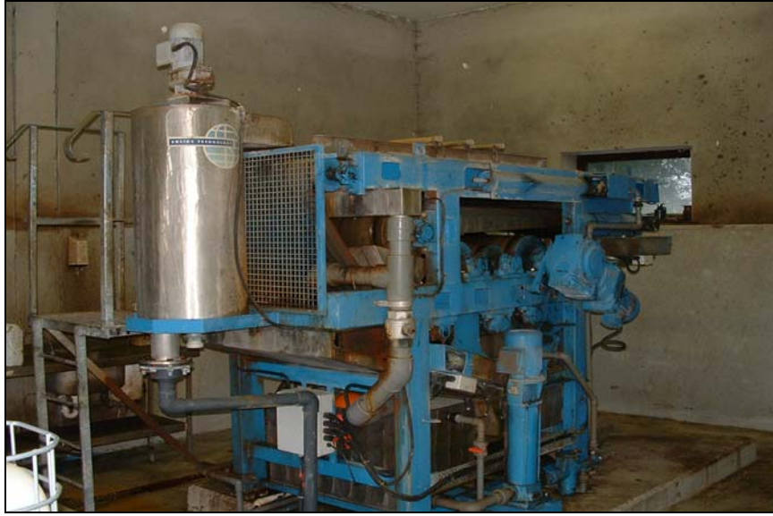
Photograph 3.9 - Belt Filter Press
