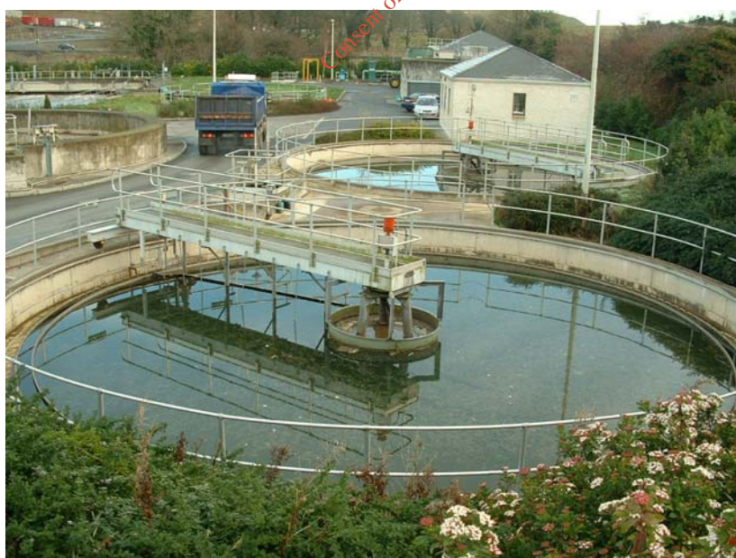
Photograph 3.6 – Final Settling Tanks
