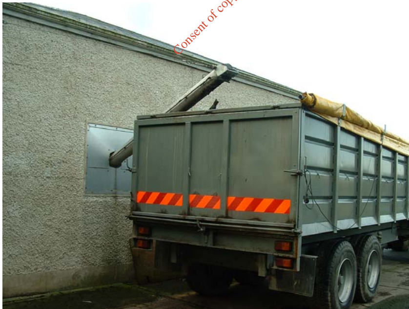
Photograph 3.10 – Screw conveyor discharging dewatered sludge to a tractor trailer
