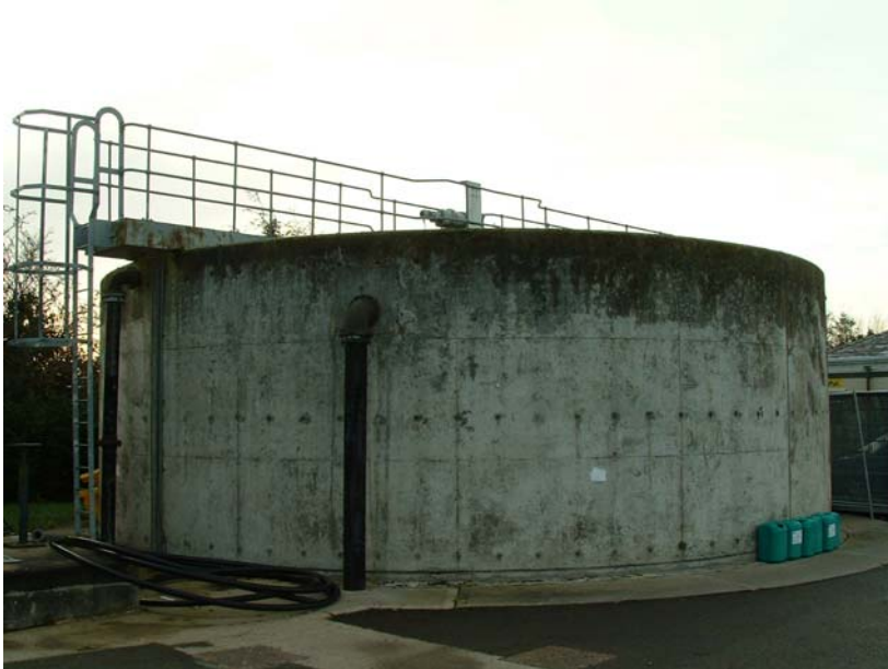
Photograph 3.8 – Picket Fence Thickener
