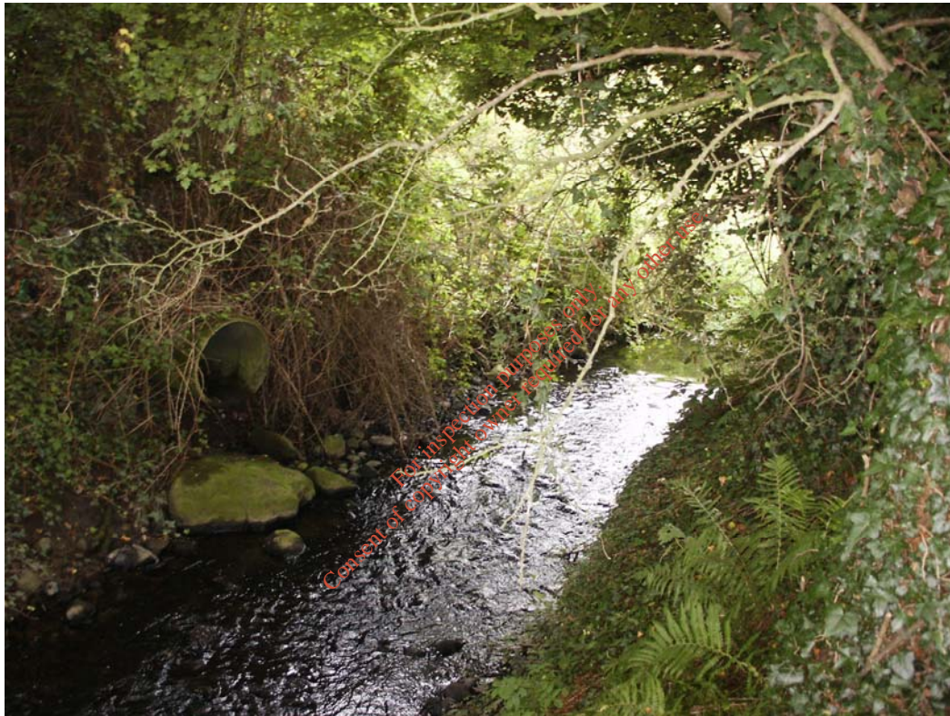
Photograph 8.3 – View of river immediately downstream of the outfall pipe.
