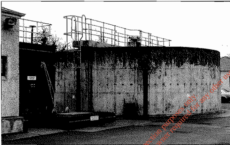
Fig. 2.07 – Sludge Thickener
