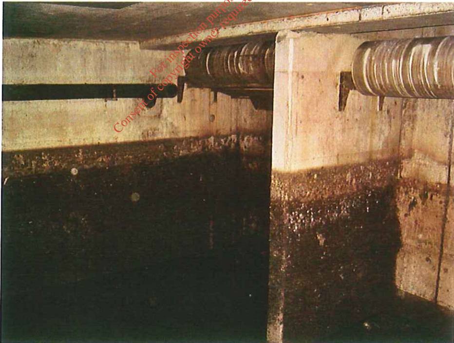
Fig. 4.20 Photo 5 – Large tipping buckets in Cell 3
