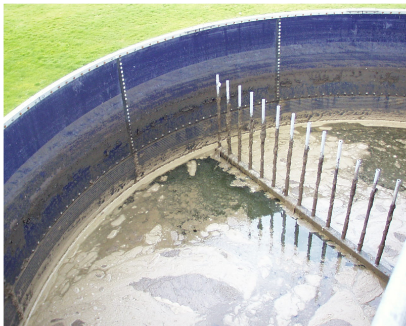
Figure 2.9 Picket fence thickener
