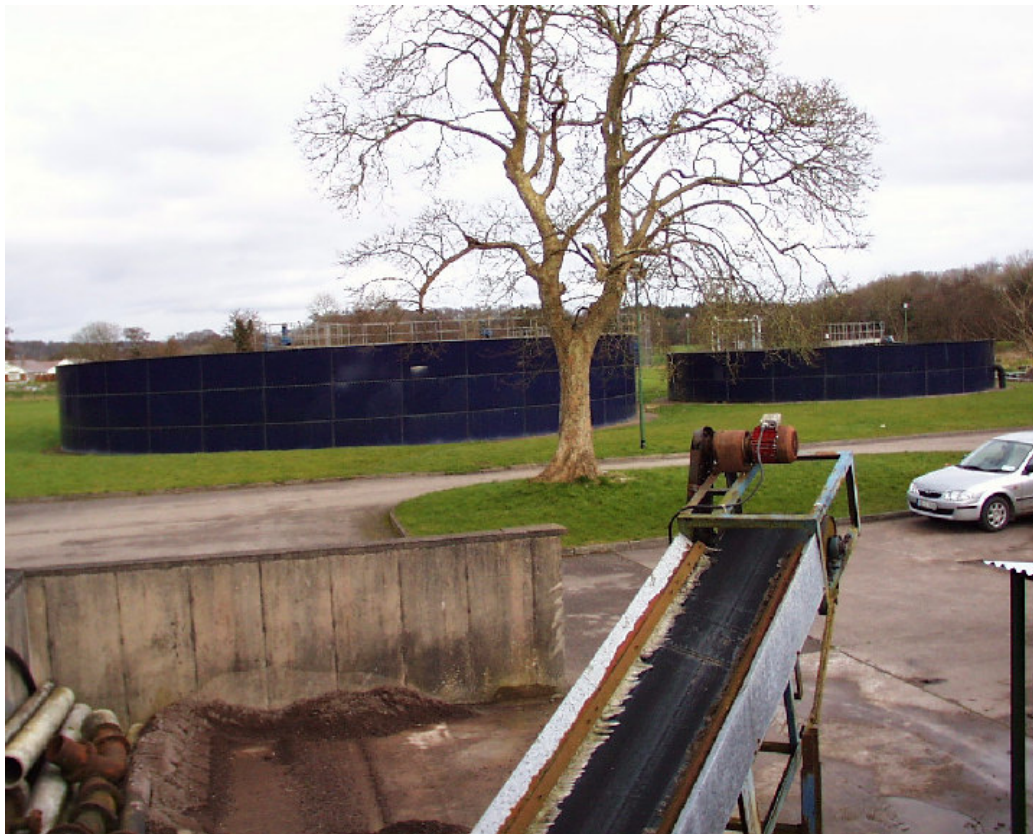
Figure 2.5 Aeration and Clarifier Tanks
