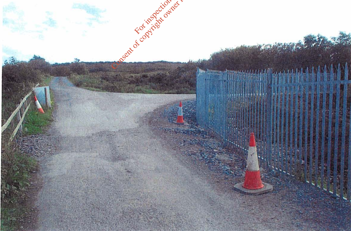
Photo G5.6 Leaving the site to the south
