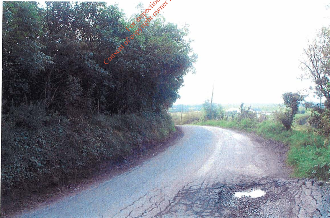
Photo G5.10 First bend (northwards) before resurfacing
