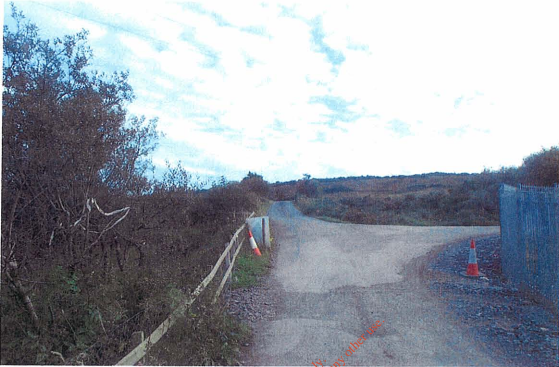
Photo G5.5 Leaving the site to the south
