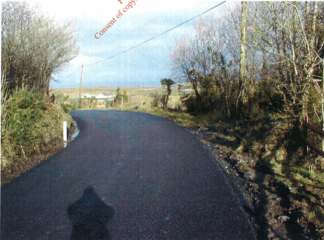
Plate 18.3 Road Integrity Has Been Improved At This Point
