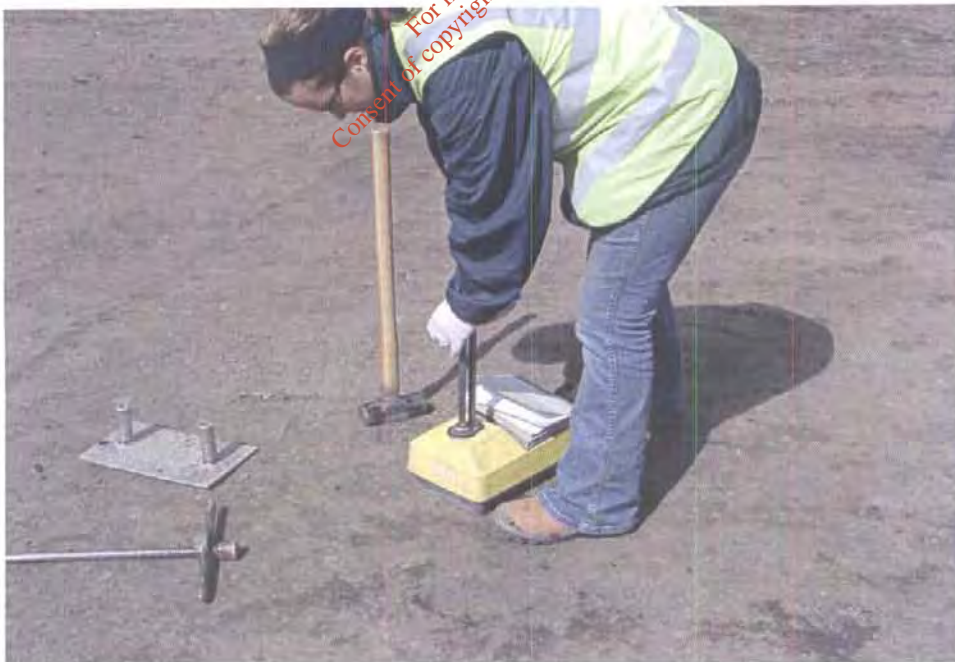
Plate 3.4.6: Testing the Clay Liner after Construction of the Cell
