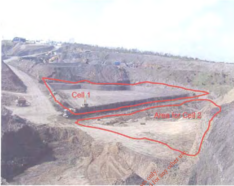
Plate 3.4.1: Engineered Cells June 2003
