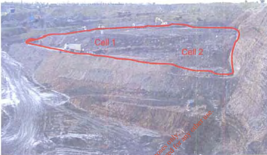
Plate 3.4.4: Engineered Cells December 2005
