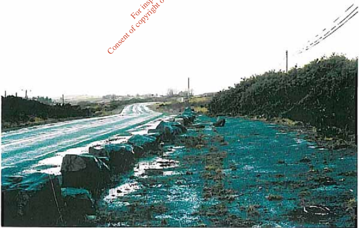
Plate 2. Verges along the R311 in the eastern sector of the survey area are wide, and in places are hardcore or gravel. View is of section of road between Derrinumeera and Cartron.
