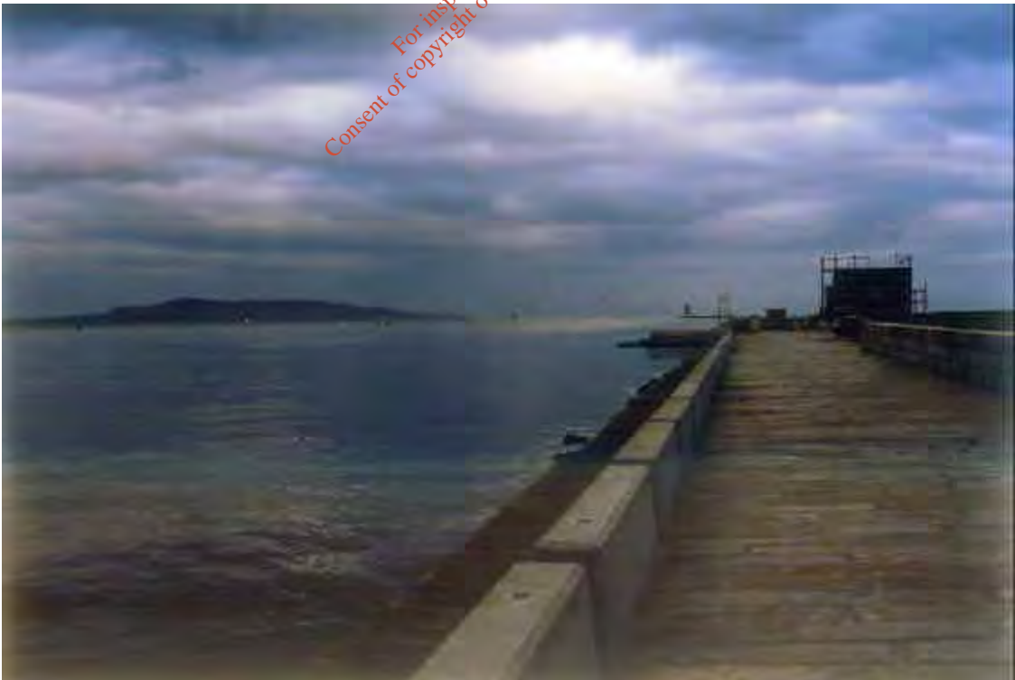
9. The Pumping Station and the South Bull - View East.
