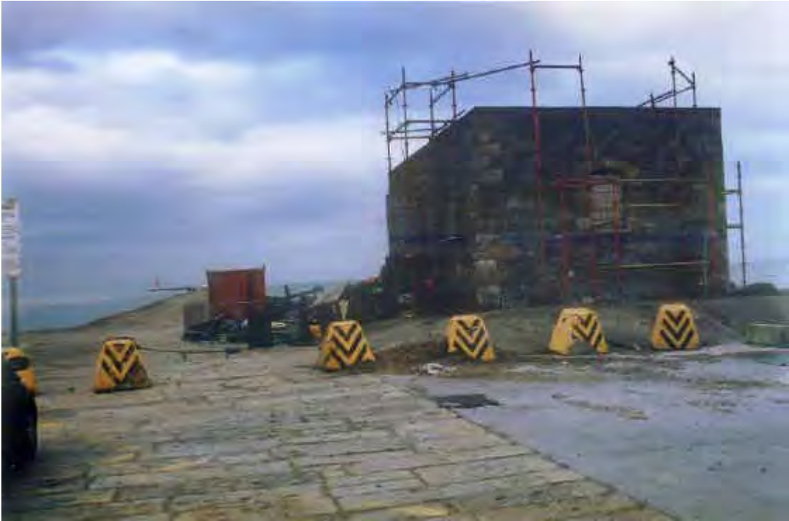
8. The Pumping Pool - View East.
