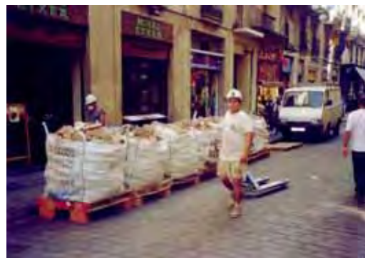
Source separation of recyclable C&D waste
