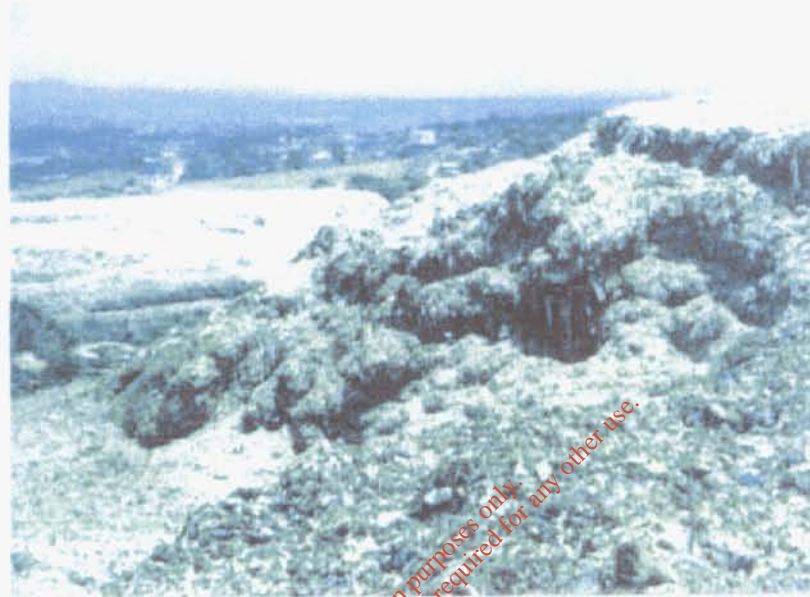
The picture above shows the situation in August 2000 about 4 weeks after the failure, when we arrived at the place to conduct a first forensic analysis. The rescue works were suspended close before. The view falls from the crest of the remaining slope over the shell-shaped failure area.
