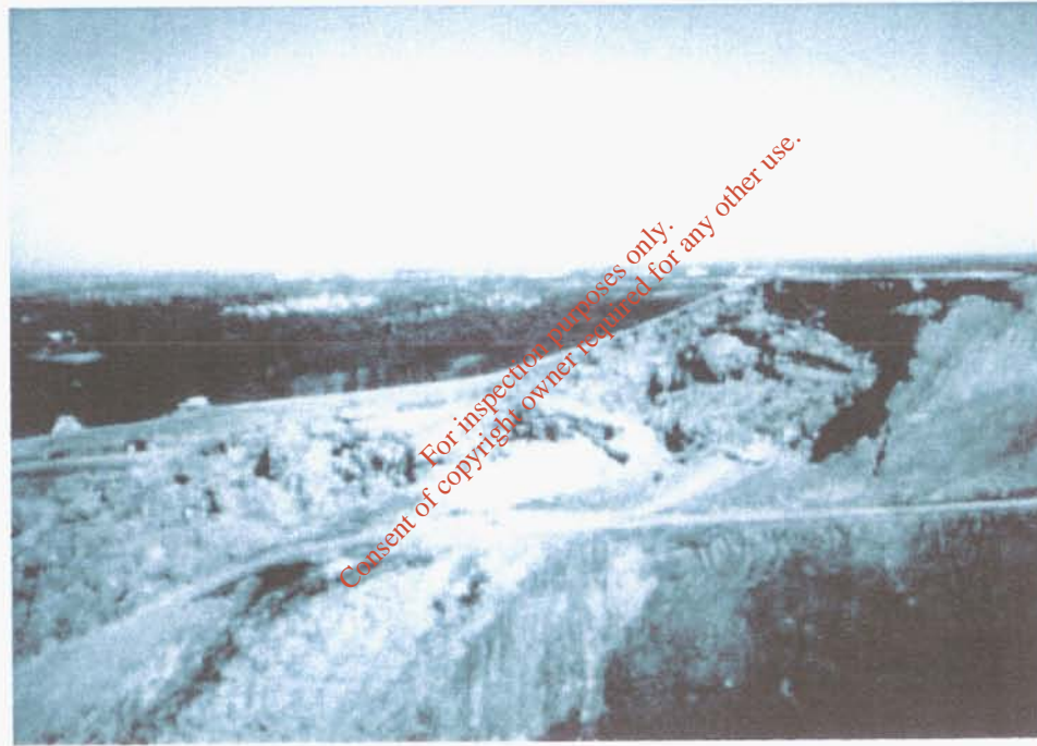
shell-shaped failure area
