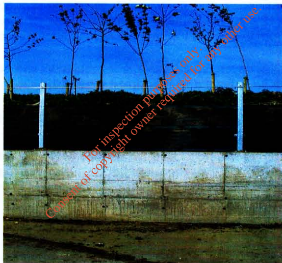
Plate 8 Wall and Earthen Boundary Surrounding the Composting Slab
