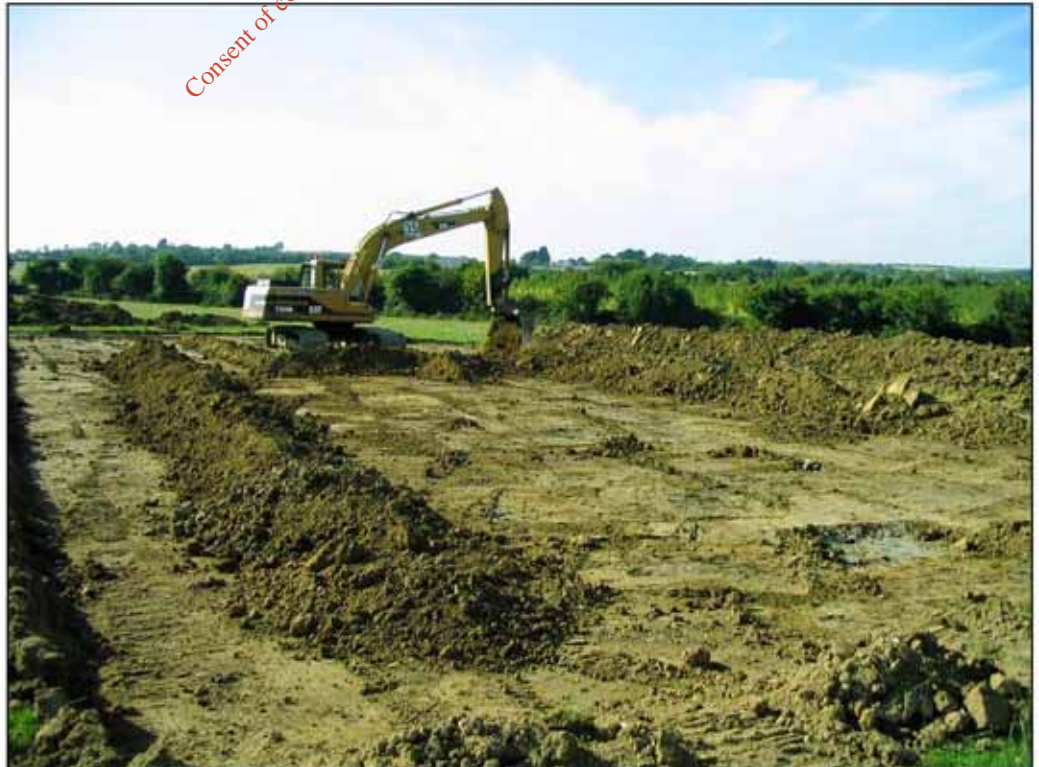
Plate 2 The stripping of Trench 4
