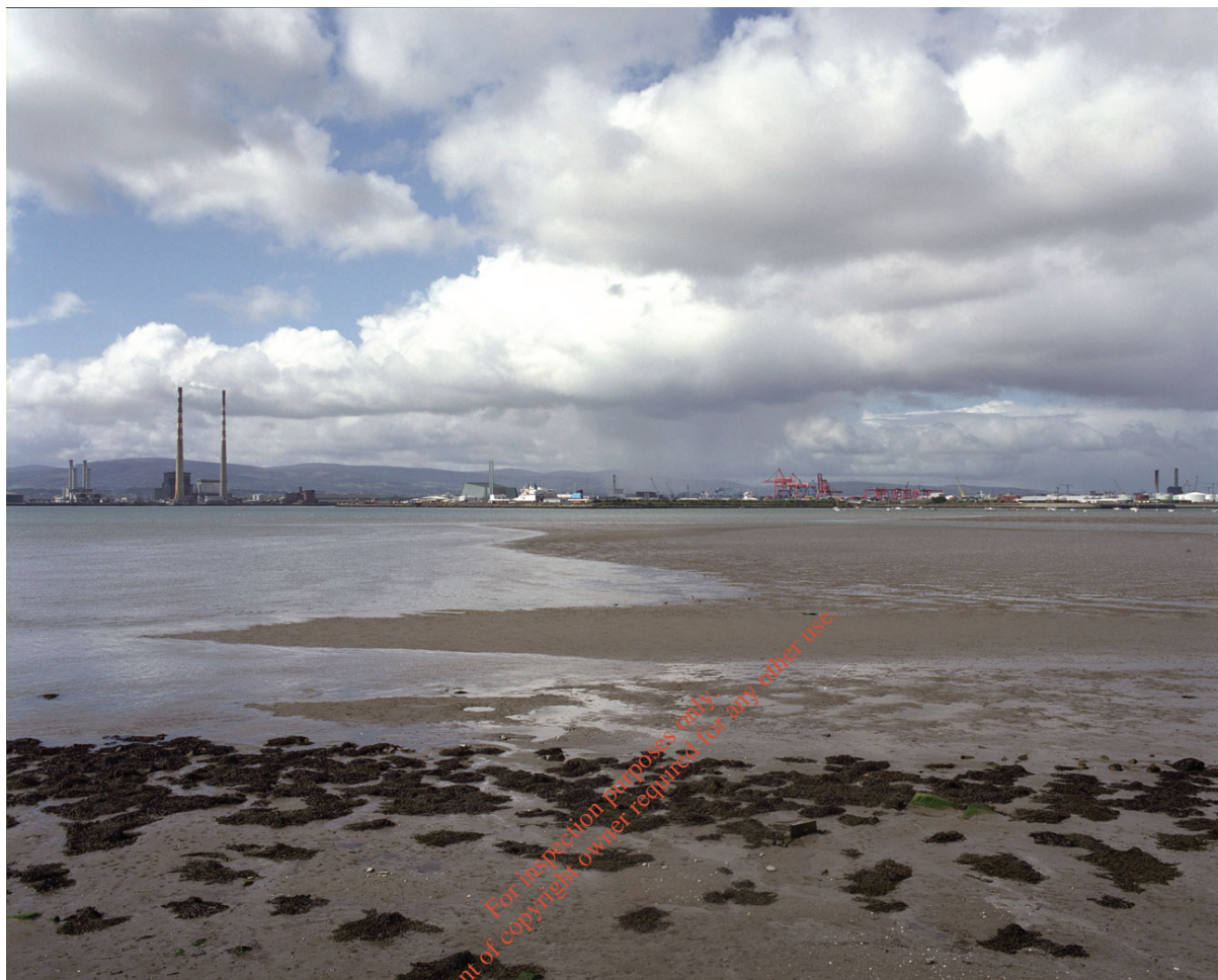
Figure 8 (Photomontage Viewpoint 7 of EIS) – an open view south from Clontarf with the twin ESB – Power Generating Station stacks dominating the horizon and standing as a clear landmark on the Poolbeg Peninsula
