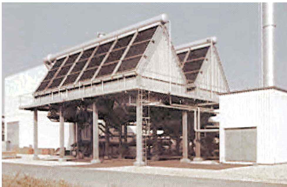
Figure 5.20 Dry cooling tower, (source: BREF document on Industrial Cooling Systems)
