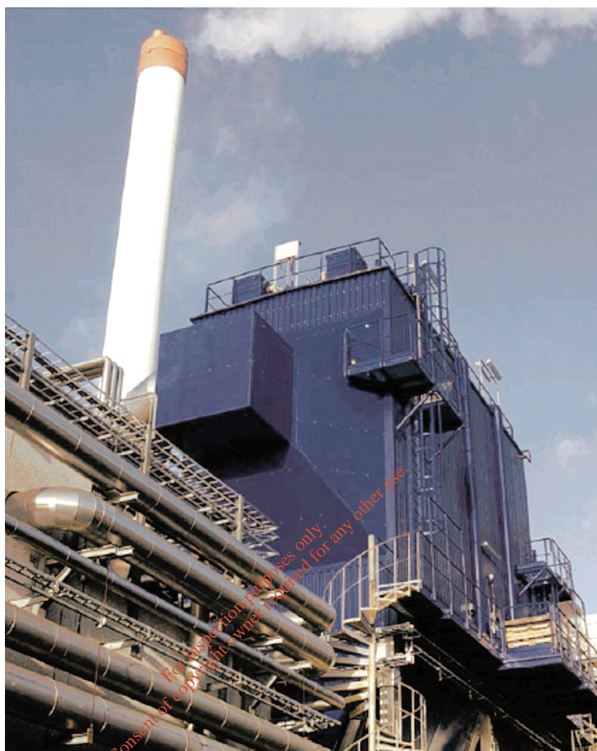
Figure 5.13 Alternative option not selected - Picture of WtE Facility without a building shell
