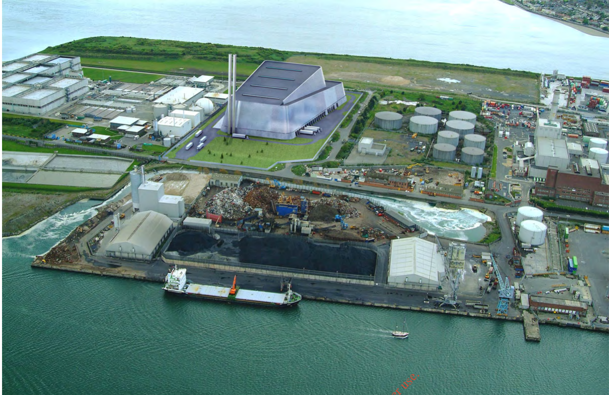
Figure 2: Aerial view of proposed Dublin Waste to Energy Facility from the North
