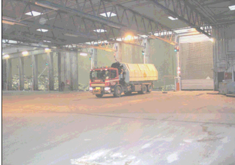
Photo 1 Waste reception hall at Elsam Odense Waste to Energy
