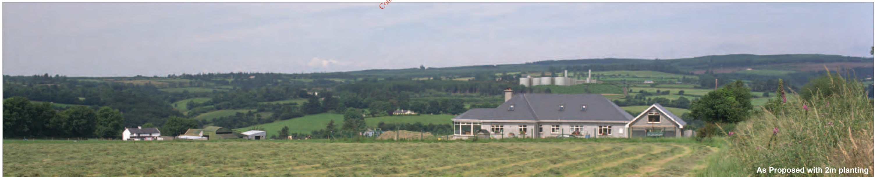
Post Construction (no mitigation)
