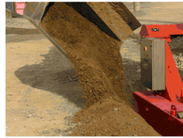
00:55 hours Backfilling around the recycling tank
