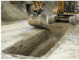
00:00 hours Digging out the pit for the recycling tank.
