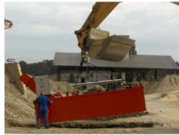
00:40 hours Setting down the recycling tank.
