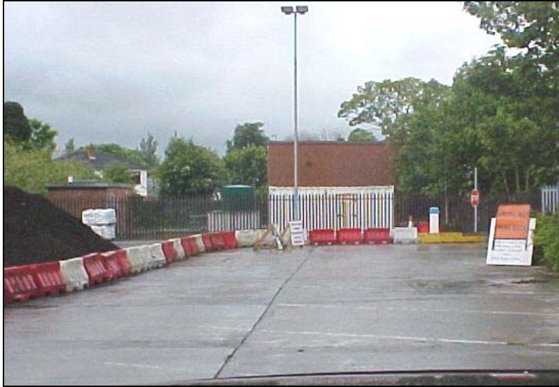
Plate D.1.b.1: User traffic is cordoned off from site operations
