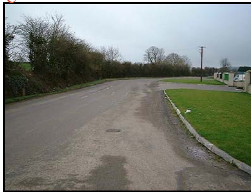
Figure 9.1.a View of Lacken Road
