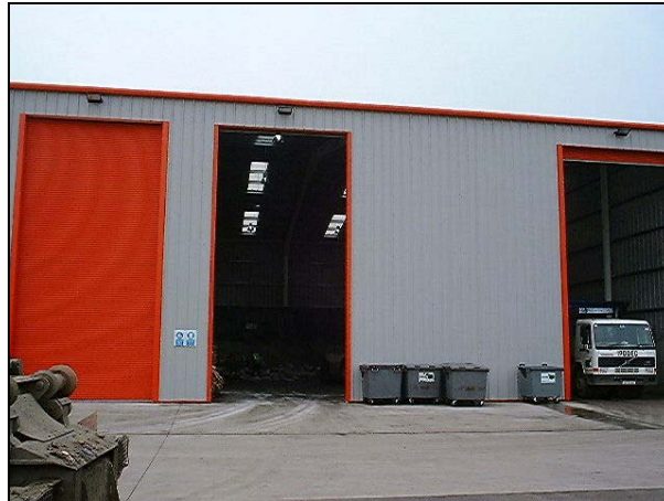
Figure 2.7.10.a Access Doors to Materials Handling & Recycling Building
