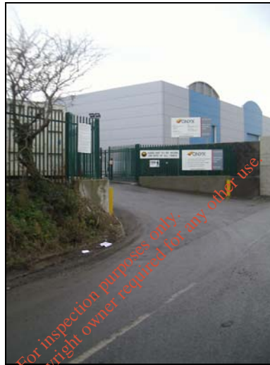
Figure 2.7.2.a. Green Road Site Entrance
