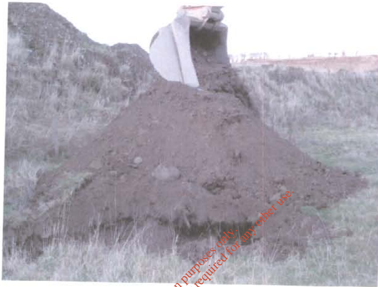
Photoview 4. Trial Pit 32 containing clean soils (no imported wastes apparent)
