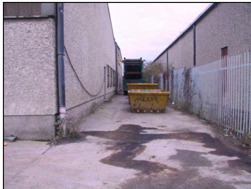
Photo Point 16 – side back entrance of proposed warehouse
