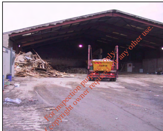
Photo Point 11 – Existing warehouse
