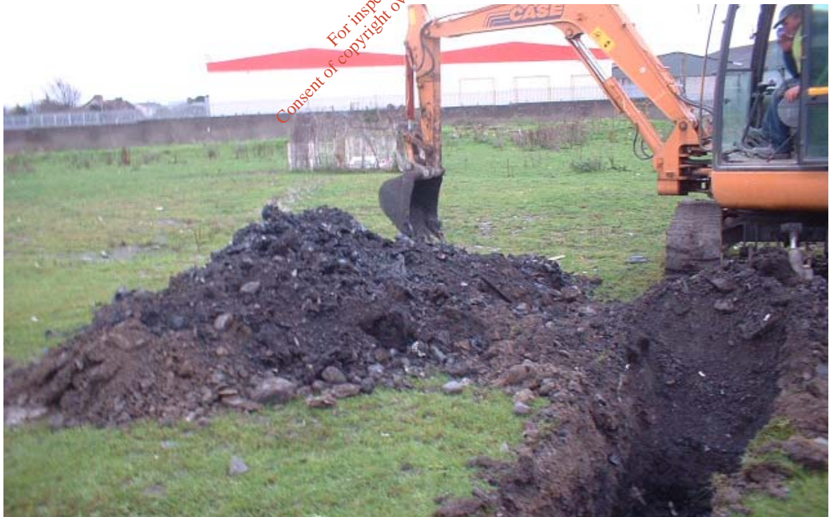
Plate 12 Trial Pit 6 Fill Material
