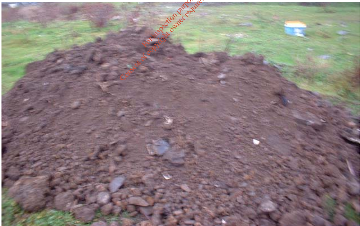
Plate 2 Trial Pit 1 Fill Material
