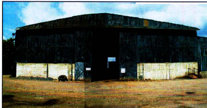
Plate 1 The High Grade Fertiliser Shed
