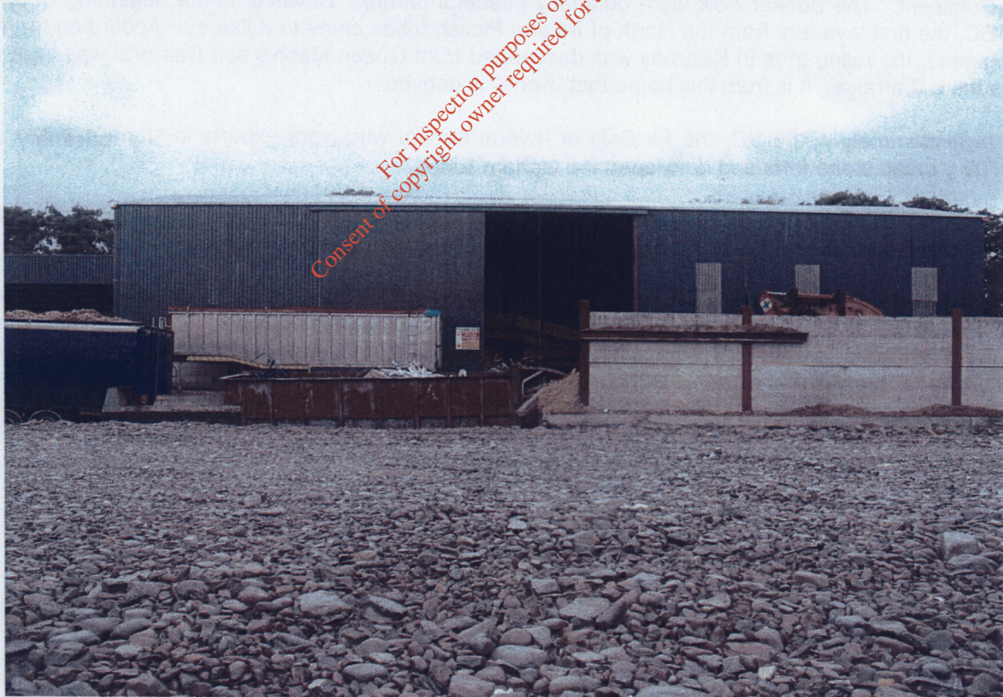
Figure 1: Area for Proposed Extension (Facing Southeast towards the Existing Building).
