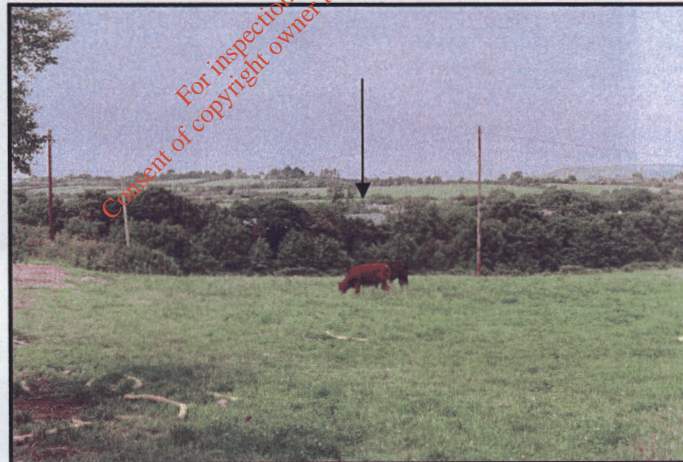
Plate 1.6 Looking northwards to the site, indicating the roof of the existing structure
