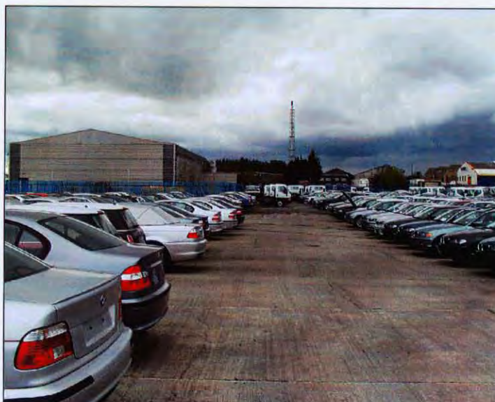
Photograph 8.1: Current site hard standing surface condition
