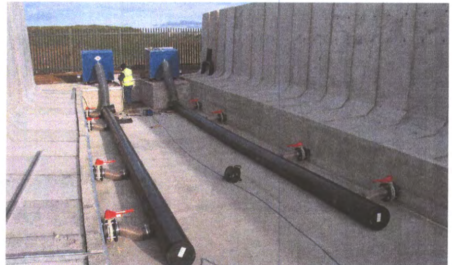
Installation of Negative Aeration System under Aerated Static Piles
