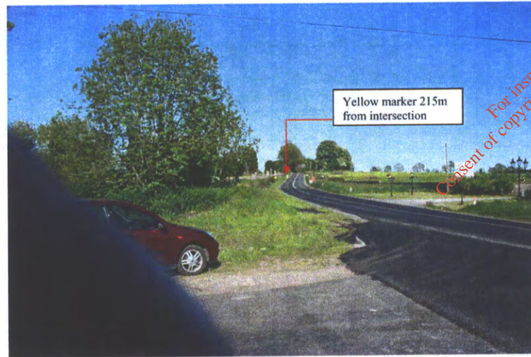
Link A2/B1 Intersection with the N6 at Pass of Kilbride. Sight line at 9 metre set back towards Kinnegad along Link B1.
