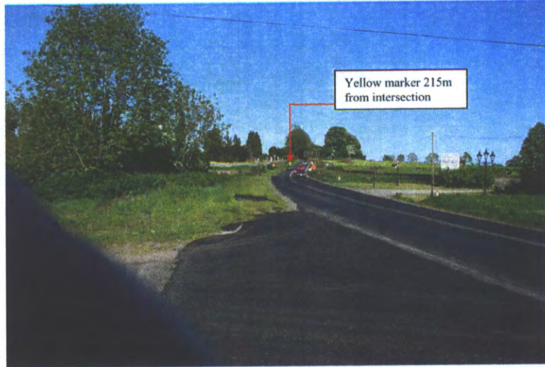
Link A2/B1 Intersection with the N6 at Pass of Kilbride. Sight line at 4.5 metre set back towards Kinnegad along Link B1.
