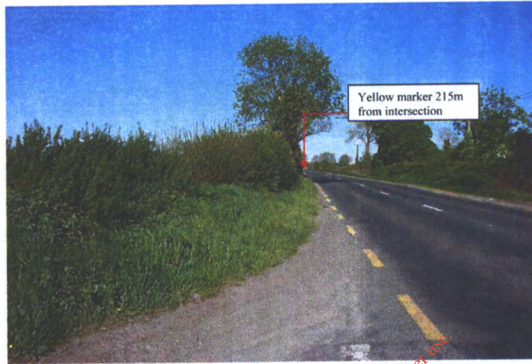
Link C/B1-B2 Intersection. Sight line at 2 metre set back towards Kinnegad from Link C.
