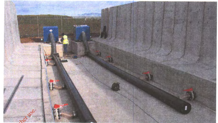
Construction of an Aerated Floor
