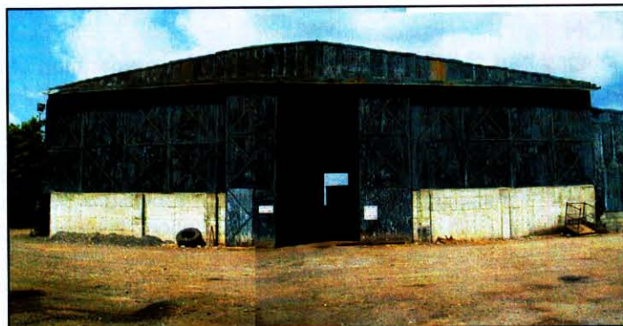
Plate 1 The High Grade Fertiliser Shed
