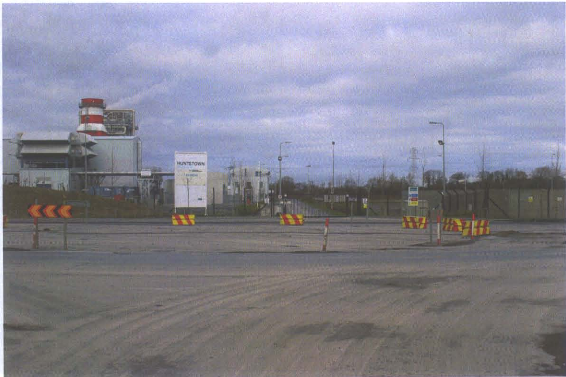
Photograph 3. The view from the quarry access road looking north is screened by the quarry and power plant.
