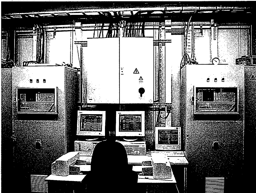
AMESA control cabinets for monitoring 2 lines simultaneously
