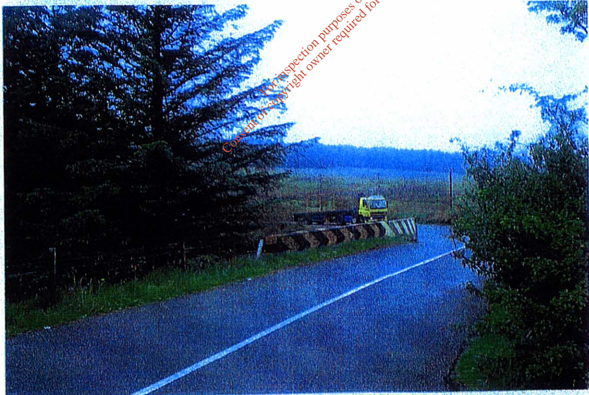
HGV approaching bridge
