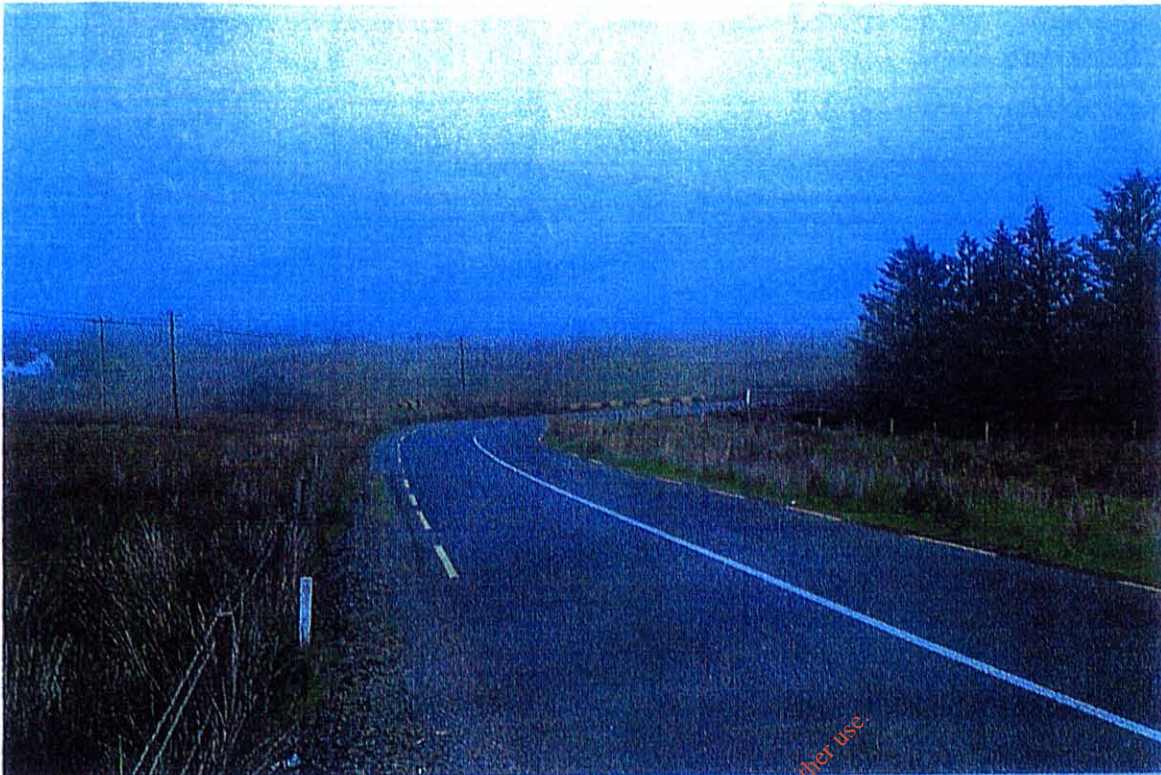
R250 traveling back from Fintown to Site. Bridge with signage
