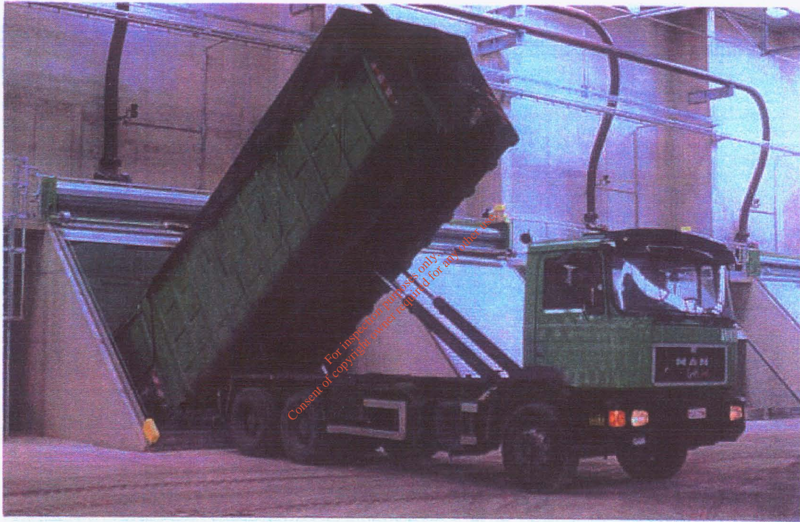
Figure 2.3 Waste Acceptance Hall of Similar Plant in Belgium
