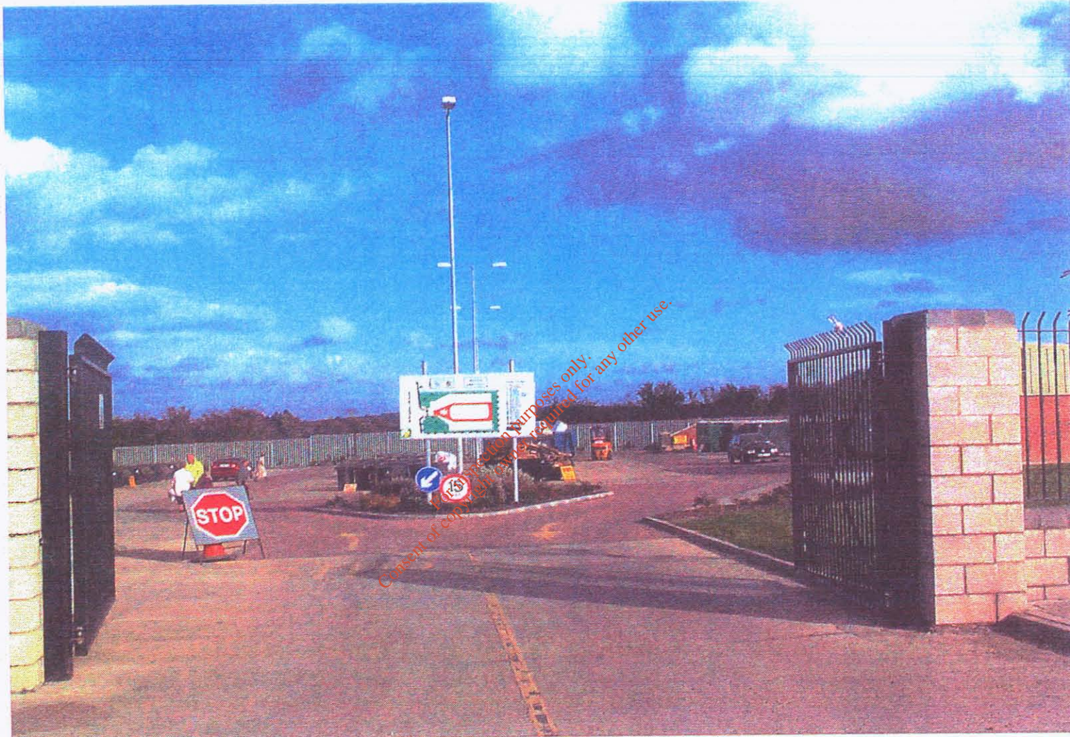
Figure 2.1 – Photograph of Navan Recycling Park
