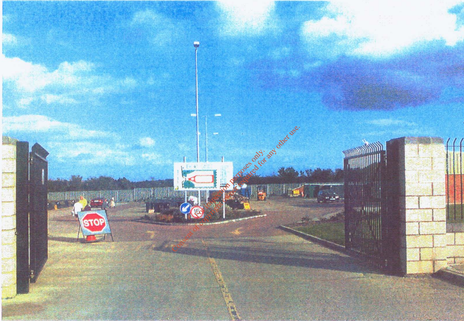
Figure 2.2 – Photograph of Navan Recycling Park
