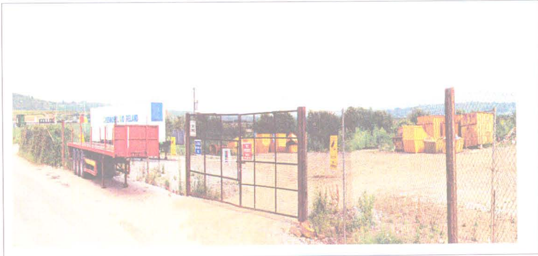
Existing Site Entrance
