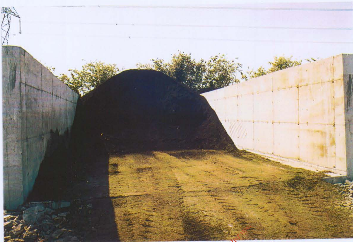
Photograph 9. Compost stored in one of the bays in the reception area
