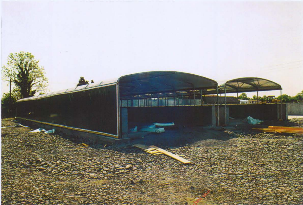
Photograph 7. 2 of the tunnels being constructed
