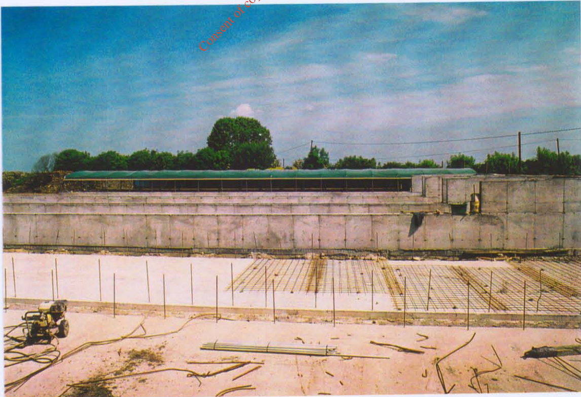
Photograph 8. Construction of the concrete base of more of the tunnels.
