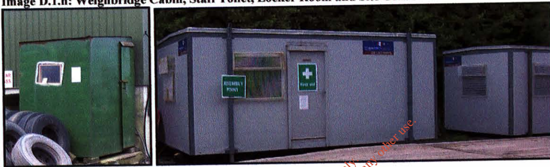
Image D.1.n: Weighbridge Cabin, Staff Toilet, Locker Room and Site Office
