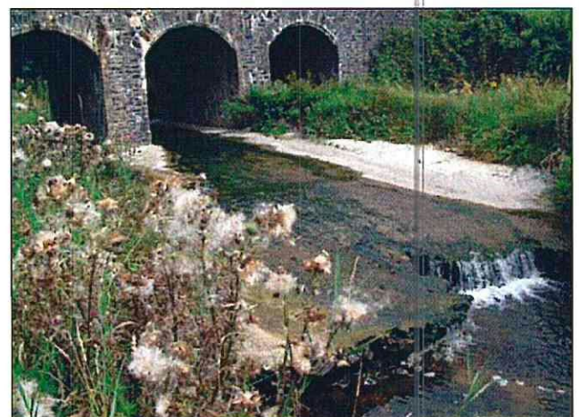
Apron/scour slab inaccessible on its downstream end to fish life because of the extent of perching and impassable due to a combination of excessive water velocity and lack of water depth across its surface.
