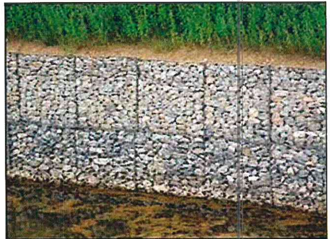
Visually unsightly stone filled gabion baskets.
