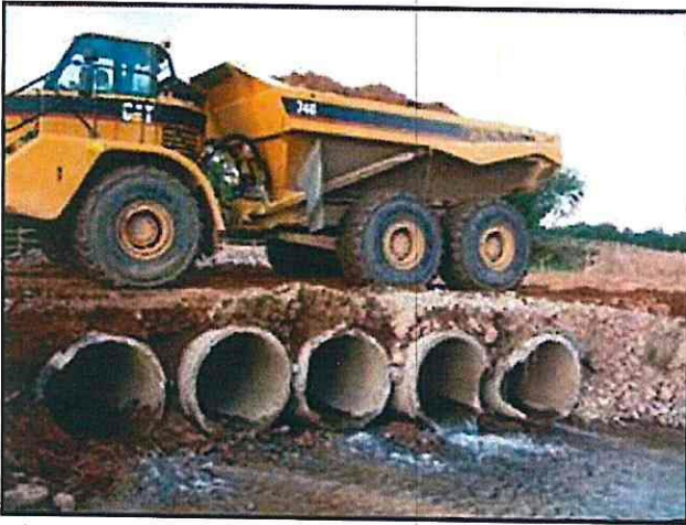
The same temporary crossing location as shown on the previous page, but with a laden dumper dislodging and causing loss of cover material to waters.
