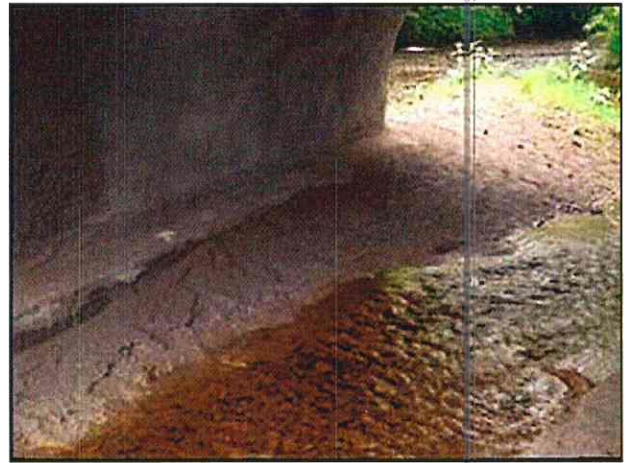
Guniting rebound on a stream bed where no precautions were taken to prevent its entry to waters. Rebound having a pH >11.5 would have entered the actively flowing stream with dire environmental consequences.
