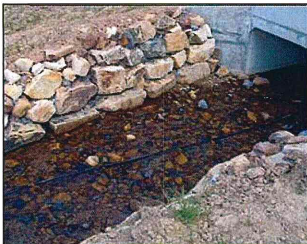
An embedded box culvert sized to match existing stream profile.
