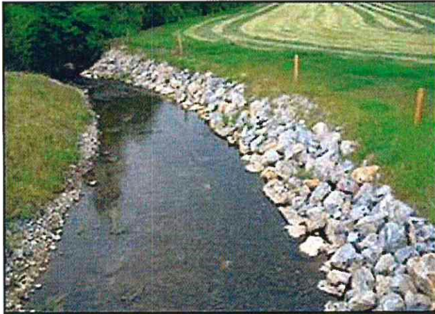
The boulders in these bank protection works are not large enough, not sunken below stream bed level and likely to be undercut and dislodged in a storm event.
