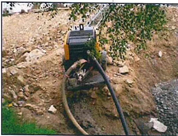
Drip tray is undersized, dangerously positioned and leaking oil. Unacceptable practice.
