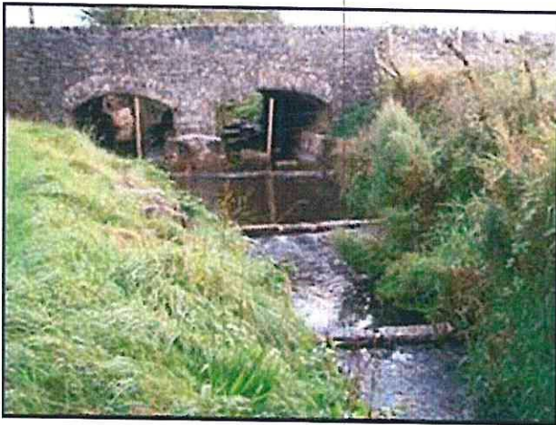
Low level stone weirs installed on a salmonid nursery stream to back water the bridge apron /scour slab originally installed at too high a level.
