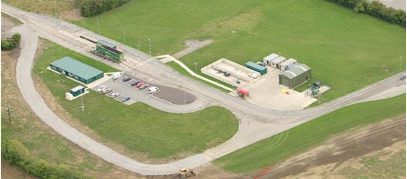
Plate 2-2: Knockharley Landfill Administration Area
