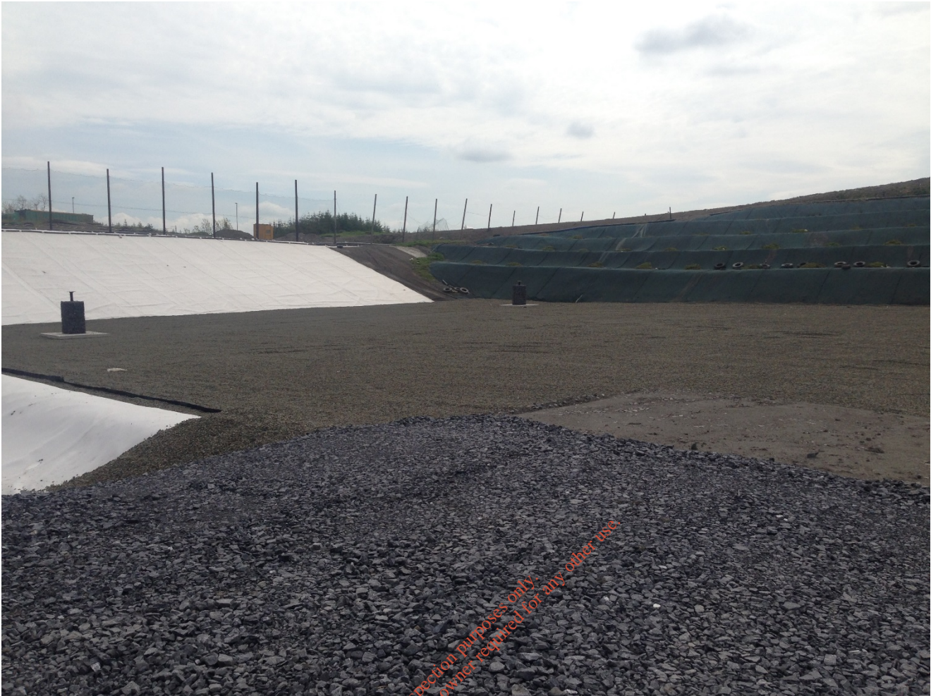
Plate 2-3: Lined cells at Knockharley Landfill
