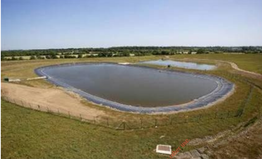
Plate 2-5: Surface Water Attenuation Pond and Wetland
